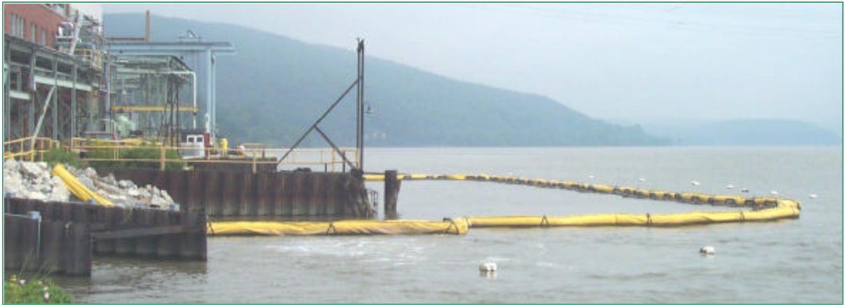
Photo 2. Lovett 1998 Gunderboom MLES™ Deployment with AirBurst™ Technology at the Lovett Generating Station, Tomkins Cove, NY.
