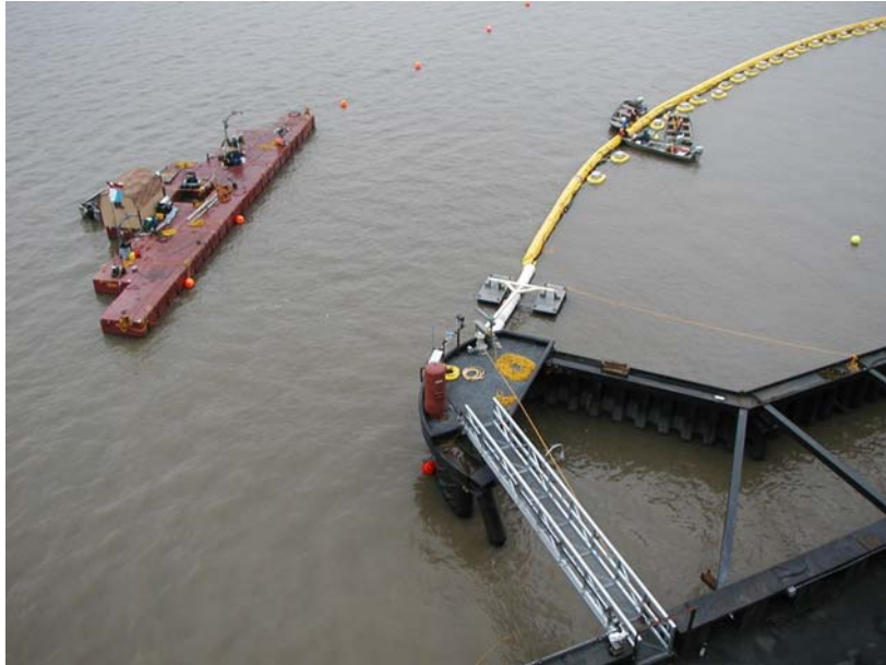
Figure 20. Divers prepare to attach anchor lines, distributing the loads by fine-tuning the lengths, and inspect the bottom seal after unreefing.
