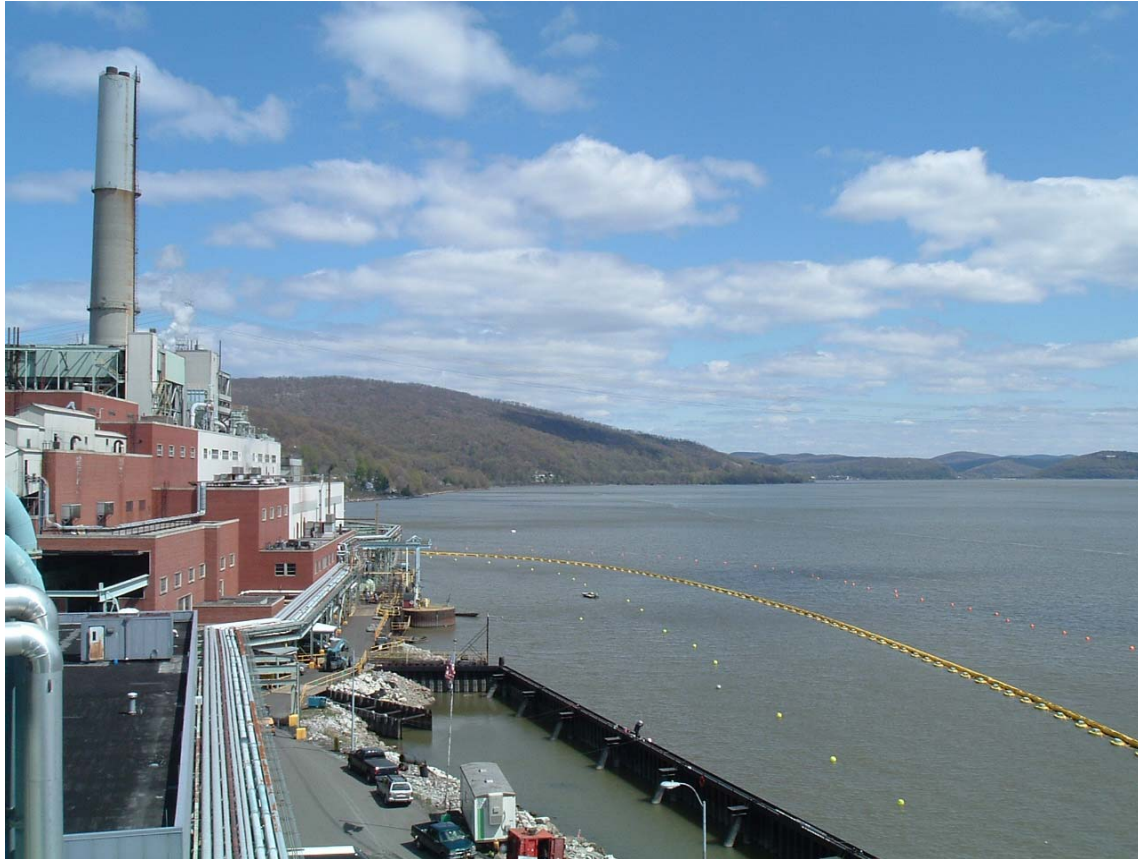
Figure 3. Photo looking northward along the Hudson River shoreline at Lovett, quickly relating the engineering drawings with a picture of the result. Here the top of the Gunderboom MLES™ can be seen as it appeared after onsite assembly and prior to attaching mooring lines from the anchors. The fabric is “reefed” to the flotation.
