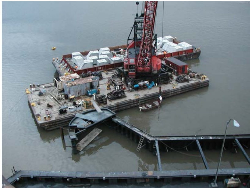
Figure 12. The North Mooring Cell is being installed at the extended Unit 5 CWP discharge channel. The system's anchors can be seen on the barge.
