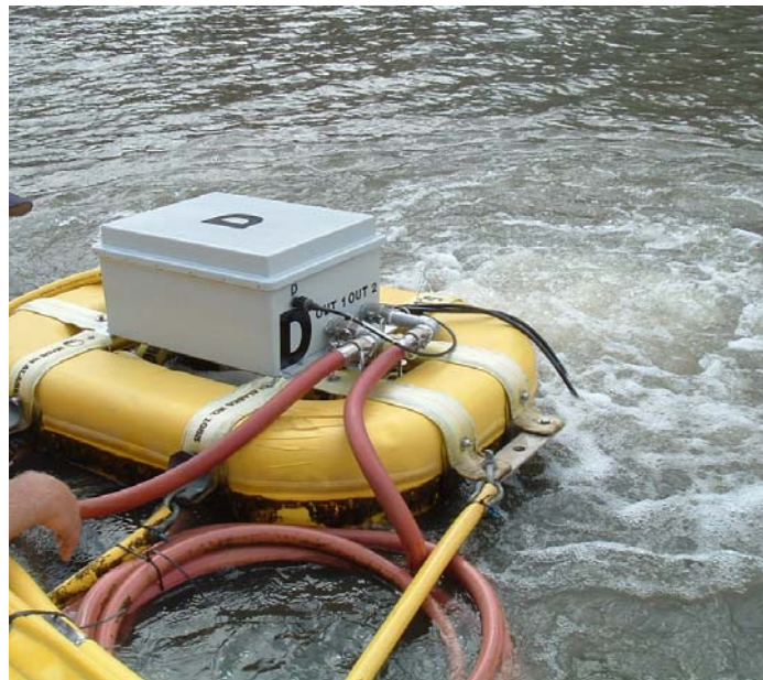
Figure 26b. Valve float box in place during AirBurst pulse.
