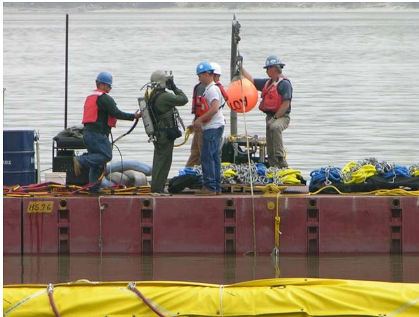
Figure 20. Divers prepare to attach anchor lines, distributing the loads by fine-tuning the lengths, and inspect the bottom seal after unreefing.
