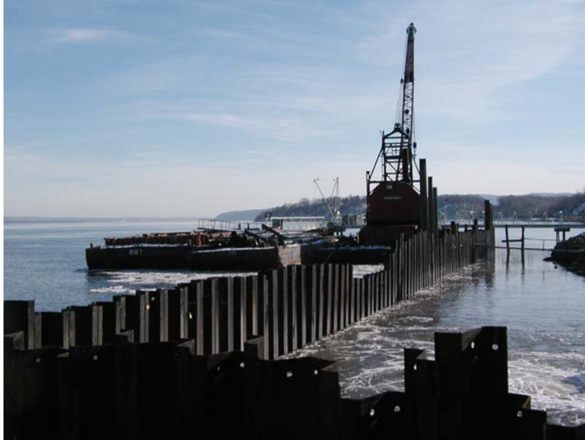
Figure 12. The North Mooring Cell is being installed at the extended Unit 5 CWP discharge channel. The system's anchors can be seen on the barge.
