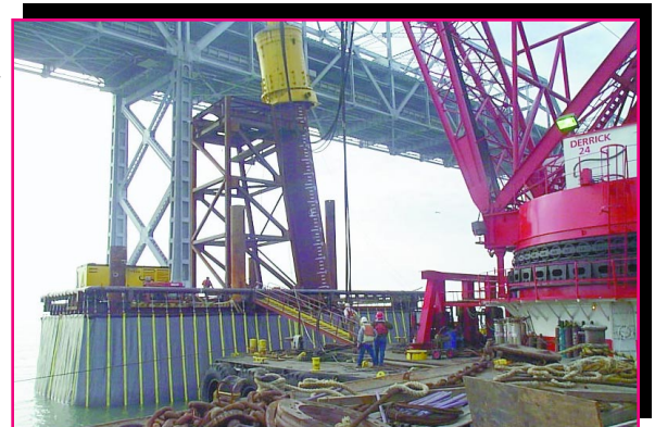
Gunderboom's sound attenuation system at work.
