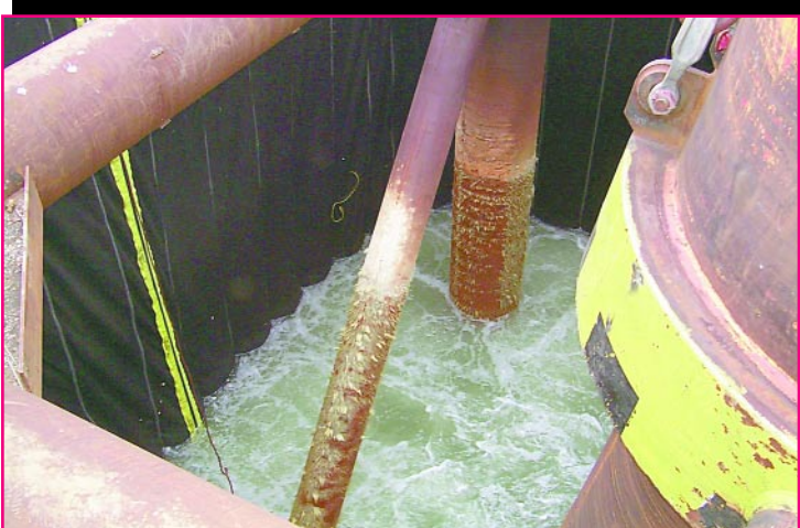
The sound attenuation curtain inside during operation with inflated absorption cells and air flux.
