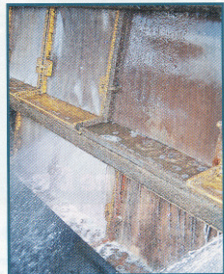
Fine-mesh screens circulated through the incoming cooling water can help exclude fish eggs and other tiny life forms, but so far have been installed on very few plants.
