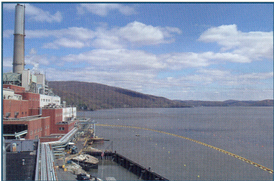
A Gunderboom Marine Life Exclusion System anchored outside the Lovett Generating Station, on the Hudson River in New York, brought about a 99 percent reduction in impingement and 82 percent reduction in entrainment. Due to new federal standards, you may begin seeing devices like this at power plants which are unable to convert to closed cooling systems.
